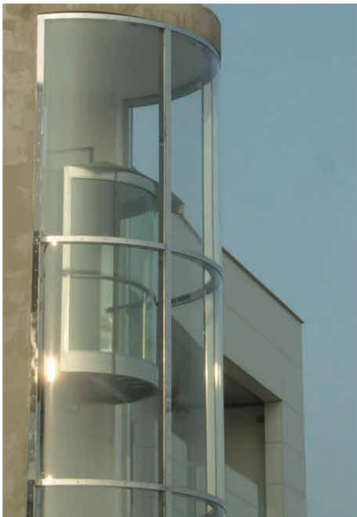
Ascensor con cabina semicircular adaptada a hueco. Lift with semicircular car adapted to shaft.
